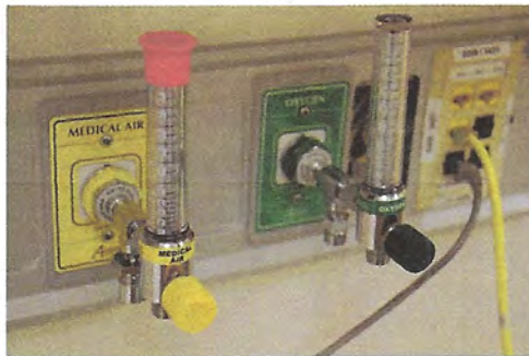
FIGURE 13.10 Color coding can be a useful technique for improving labeling on (a) receptacles and (b) connectors.
